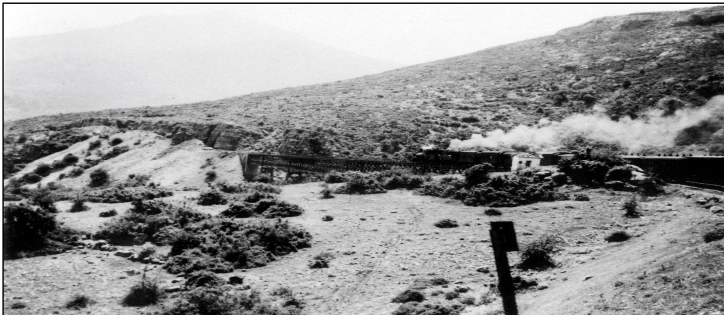
The troop train from Navplion to Kalamata - photograph taken about midday on 26 th April 1941. The train is about to cross the lattice girder viaduct at Sirtis between Achladokampos and Eleohorion villages. There were Ju 87s overhead at the time but, did not attack. There were about 50 RASC, 517 Topo and Map Depot pers and other L of C troops, plus Greeks on board. A Tank Corps major was on the footplate of the 1st engine. Photograph was taken from a window of rear carriage.
